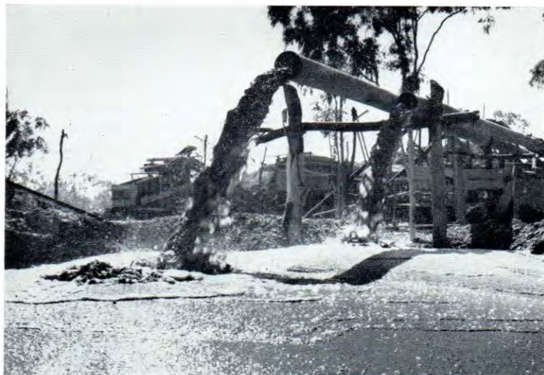
Effluent from an ore-crushing plant discharging into a freshwater river. For miles downstream the river is choked with silt.
