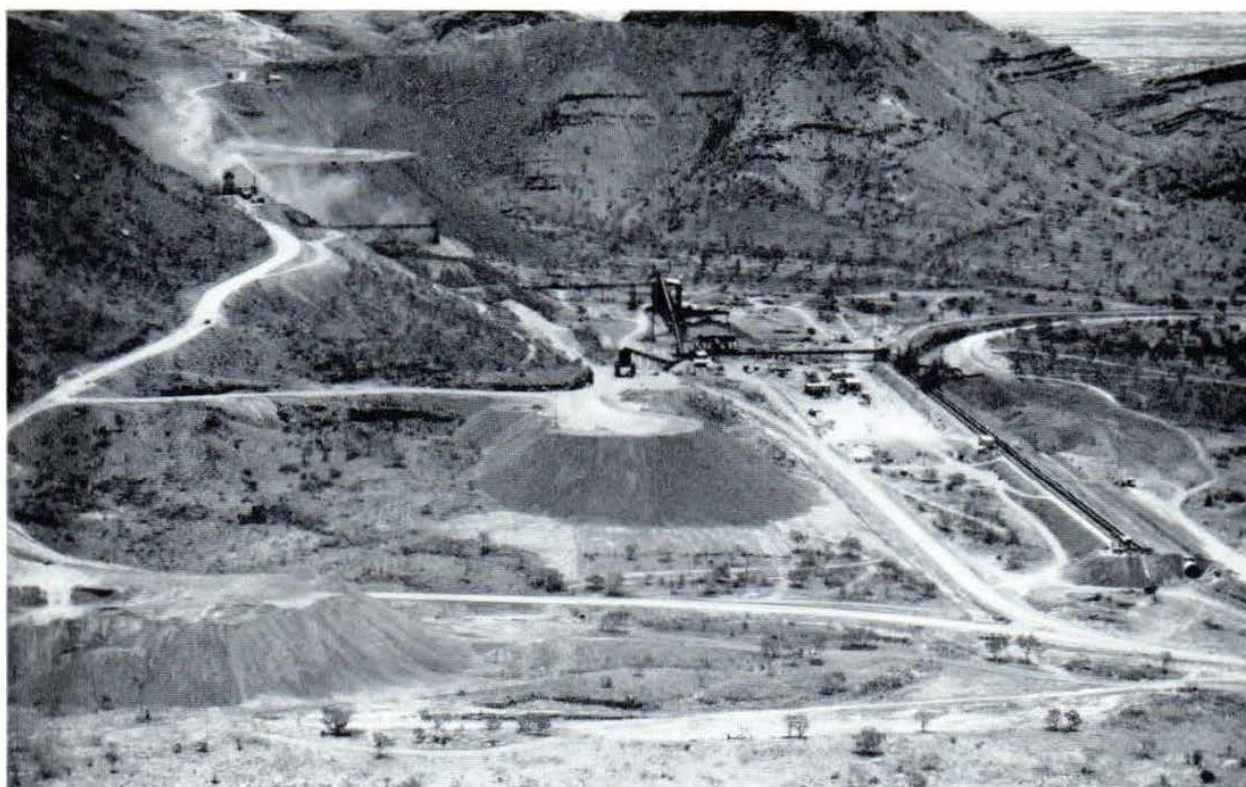
An aerial view of the treatment area at Mount Tom Price, Western Australia. One of the iron ore stockpiles is in the centre. The big building in the left background is the primary crusher. [Photo by courtesy of Hamersley Iron Pty Ltd.]
