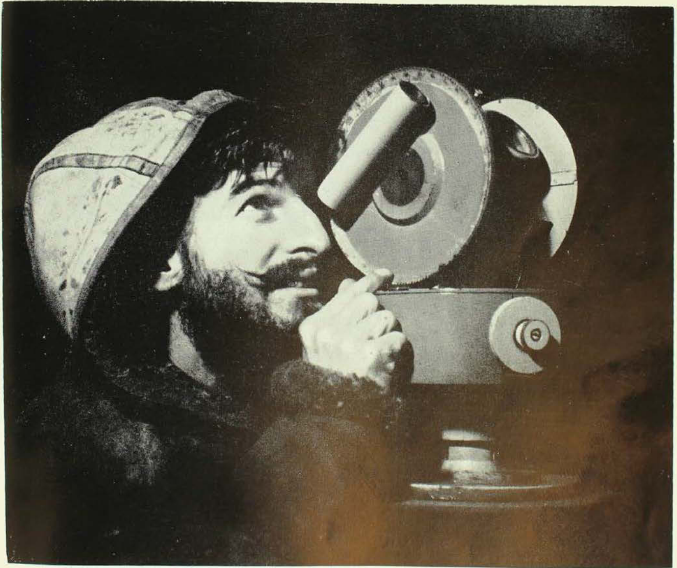
Surveying the night sky at Macquarie Island with a photo-theodolite.
