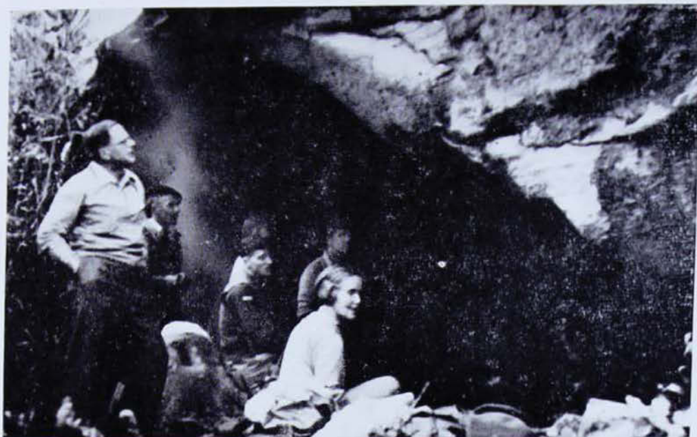
Our party inspecting another gallery at the headwaters of Cordeaux Dam.
