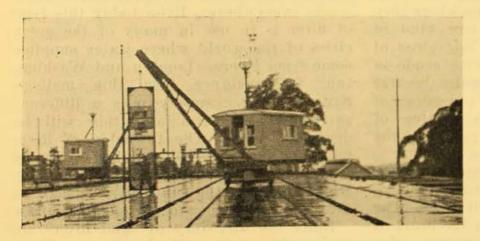
Sydney's water is purified by passing it through screens of fine wire mesh. One of these screens is seen here, hoisted from the side of the filter chamber for cleaning. An electric crane moves up and down along the side lifting the screens as required. The size of the screen may be judged by comparing it with the man's figure seen through the mesh.
