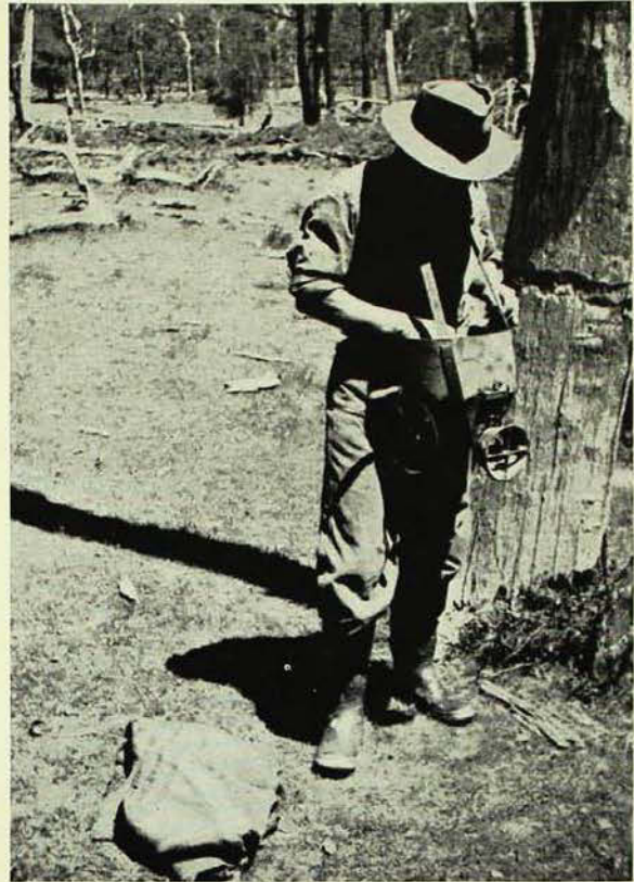
The seed broadcaster used to spread the sand and bluestone. The mixture is placed in the hopper of the machine and the handle at the side is turned while the operator walks along the area to be treated.
