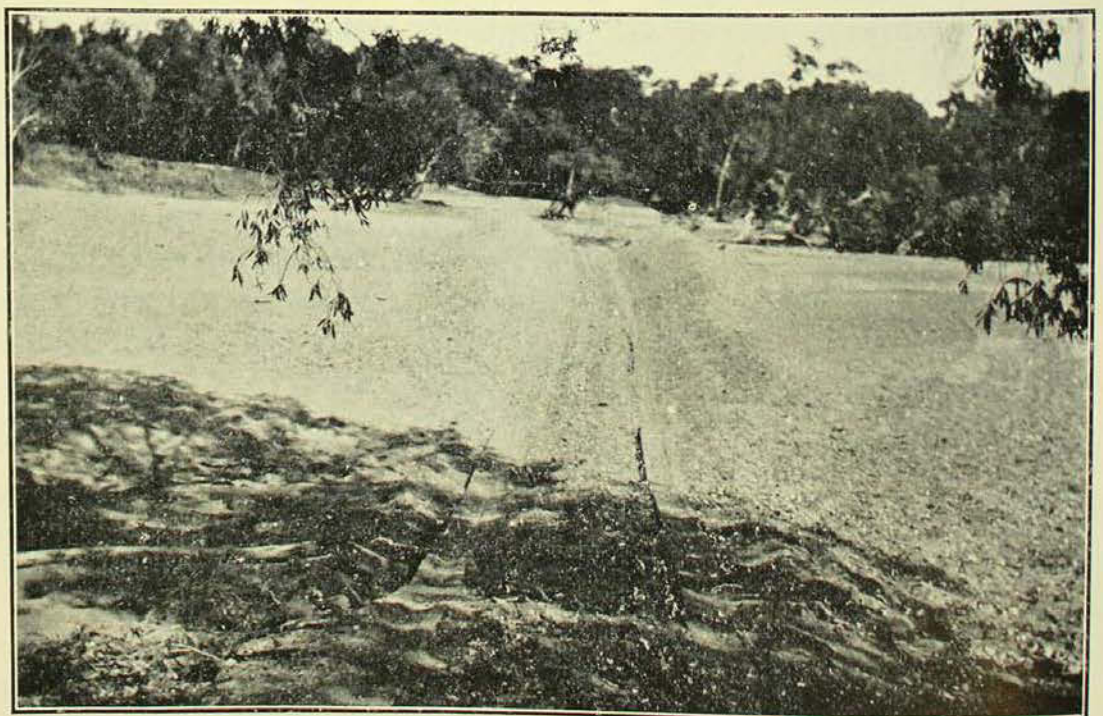
Narrow concrete strips assist the motorist in negotiating the wide sandy crossing of the Gilbert River. This river is a well-known haunt of the Estuarine Crocodile.
